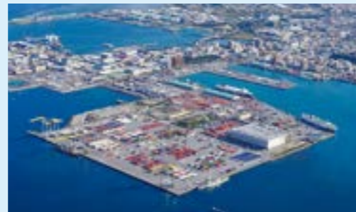
Naha International Container Terminal
