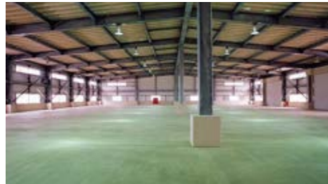
Interior of leased factory
